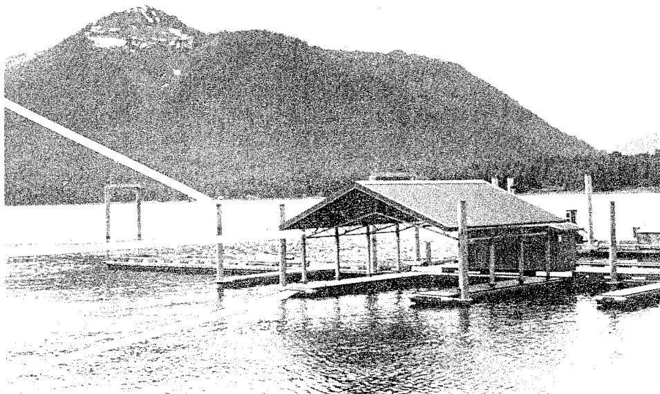
STEEL AND CONCRETE BOATHOUSE CONSTRUCTION
